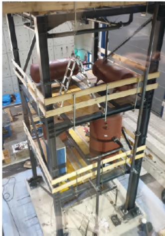
(a) Construction Phase.
